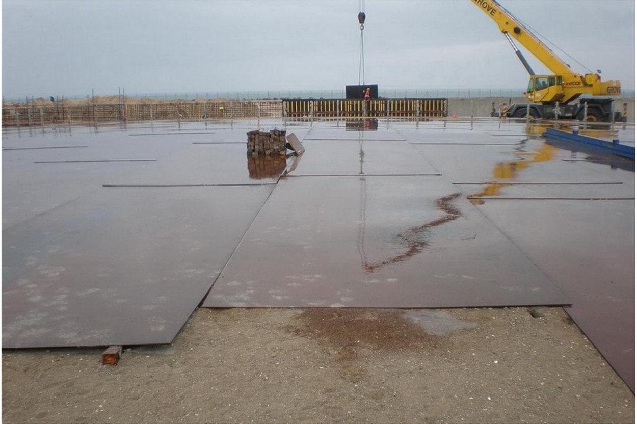
**Figure 4.4 Bottom Plate Laid on Foundation**
