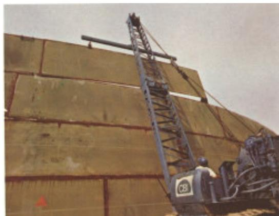
**Figure 4.8 (b) Erection of Upper Shell Course – Outside Tank**
