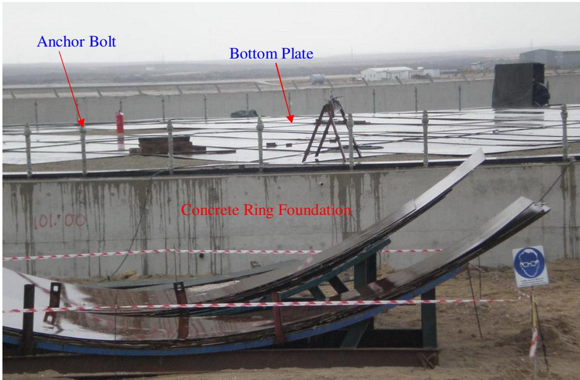
**Figure 4.2 Tank Foundation with anchor bolt installed**
