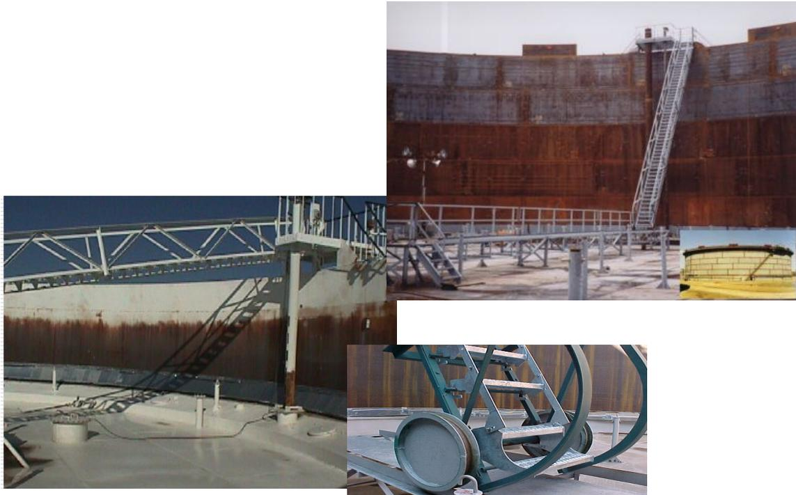
**Figure 3.28 Rolling Ladder and Gauger Platform Installed in a Floating Roof Tank**
