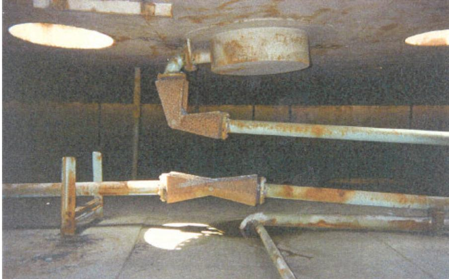
**Figure 1.26 Articulated drain pipe system installed inside the tank**
