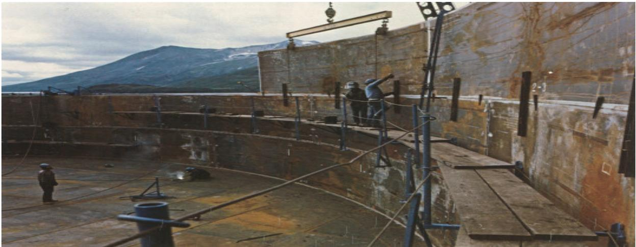
**Figure 4.8 (a) Erection of Upper Shell Course – Inside Tank**
