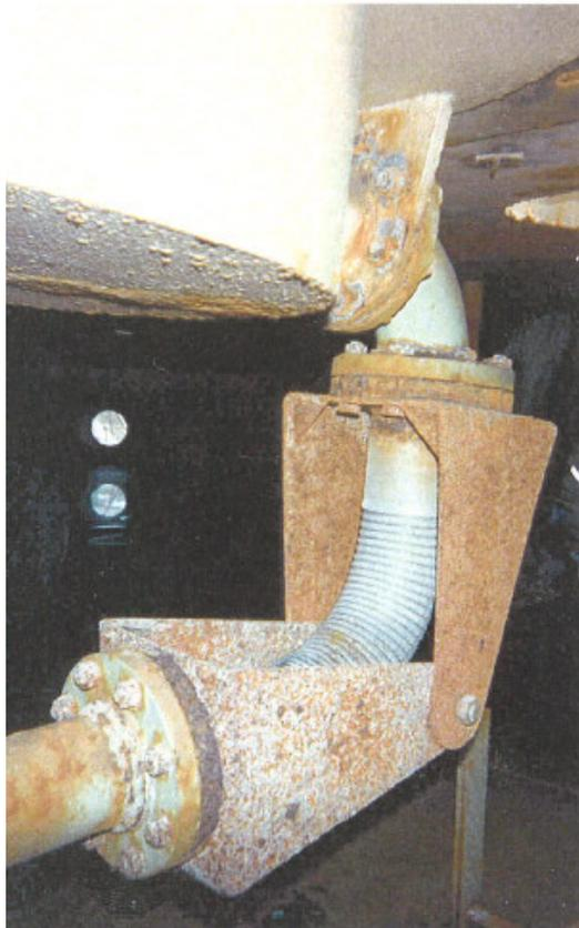
**Figure 1.27 Flexible Swing Joint**
