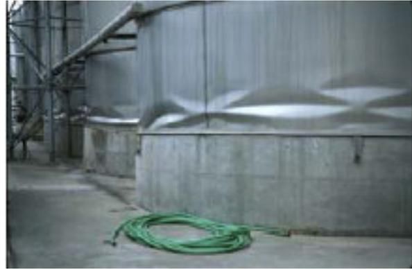
**Figure 1.17 Diamond buckling (slender tanks)**
